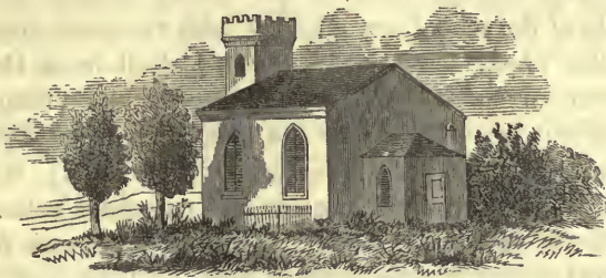
Zion Church, prior to enlargement.
